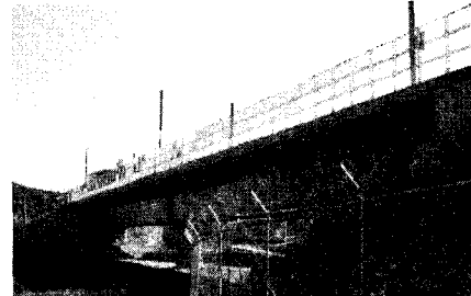
(f) High-speed railway bridge 2
