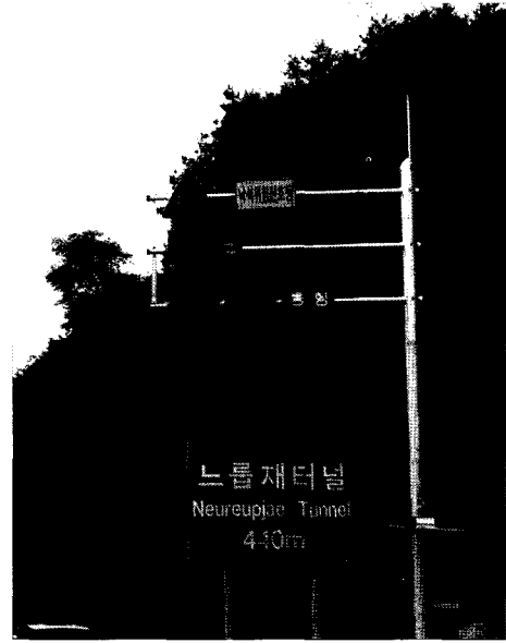
Fig. 8. Rock-fall Signal Lamp System at Neureupjae site.
