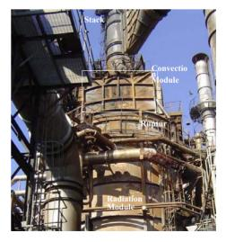
Fig. 2. Appearance of the fired prefractionator reboiler
