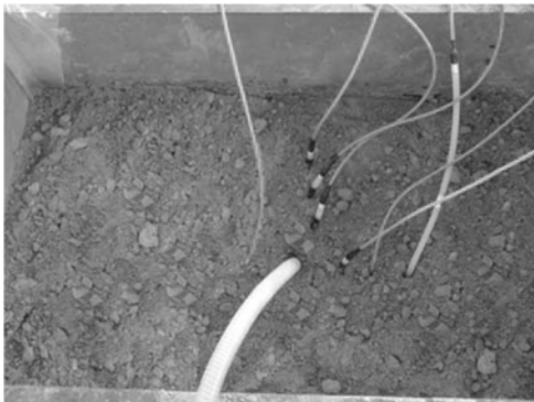
(b) PVD extraction and piezometer installation setup
