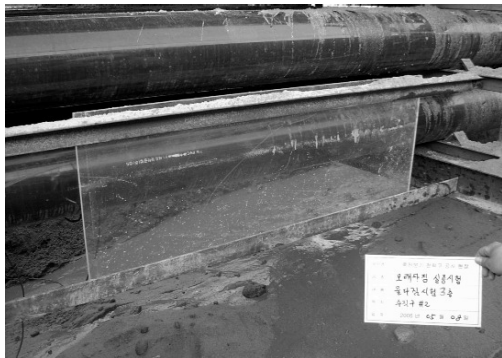
Fig. 2. Acrylic plate placed to confirm compaction by watering
