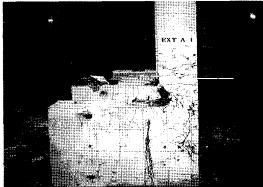
(b) Crack pattern
