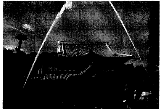
Figure 4. Operation of the water gun at main temple.
