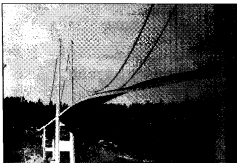
Figure 4. Vertical and torsional oscillations in Tacoma Narrows Bridge
