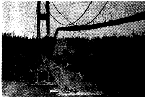
Figure 6. Bridge midsection crashing into the waters of the Tacoma Narrows, November 7, 1940
