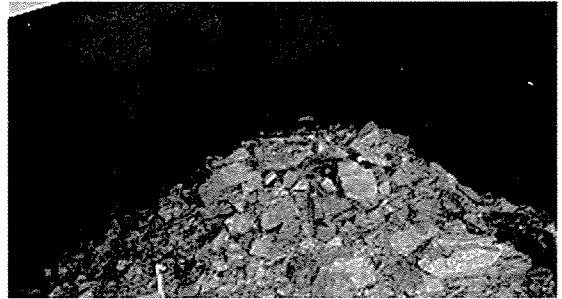
Photo 2. TBM Head부 붕락
