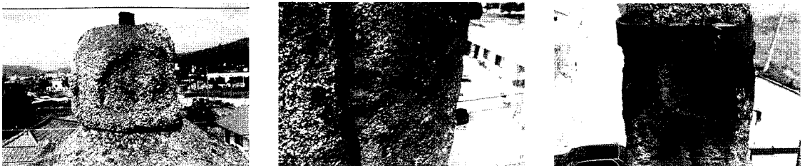
Figure 7 a. grain peel-off due to weathering at the front face b. blackening and minor crack due to weathering c. blackening by weathering product of iron band and weathering of the rock at left side
