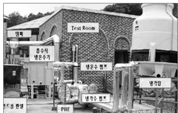
Fig. 8 Schematic diagram of MGT cogeneration system
