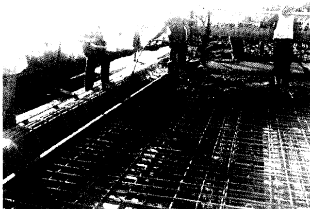
(b) Concrete consolidation
