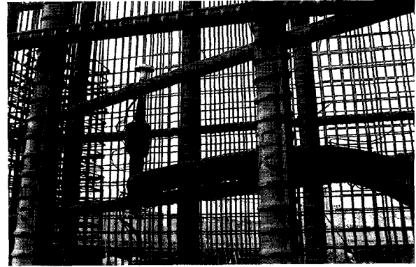
Fig. 7 Vibratin wire strain gauge installed between rebars
