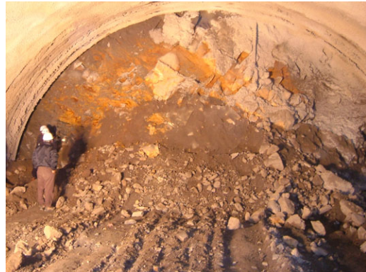
Photo 2. View of tunnel face
