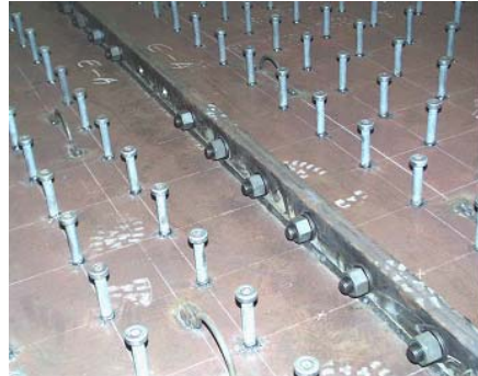
Photo1 HTB Tensile Connection (Type Eo)
