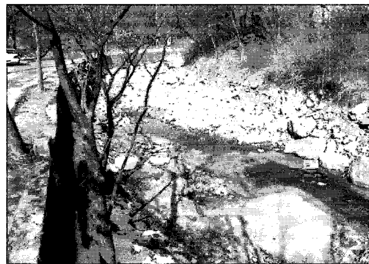
Photo 4. Streamflow Leakage Due to Bed Materials (Suamcheon, 2003)
