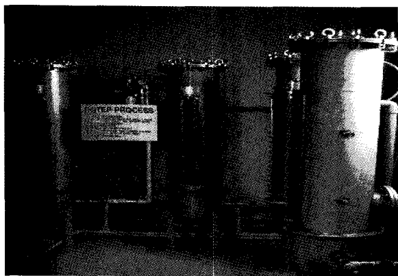
Fig. 2. Pilot plant for phosphorus treatment from farm wastewater.
