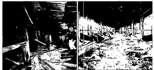
(a) burned platform and train (b) inside the burned train
