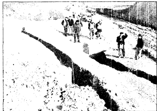
Fig. 1. Slope failure in the primary excavation stage
