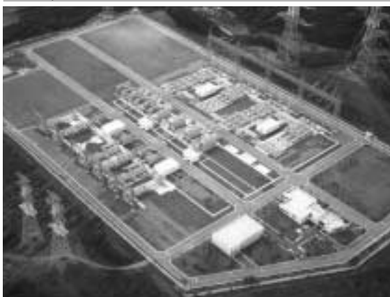
4 | 765kV ( Full GIS )
