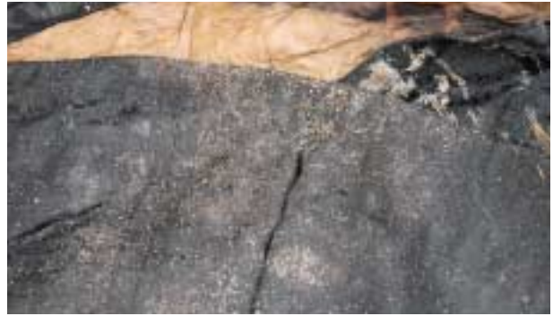
Photo 20. The damage by insect and microorganism
