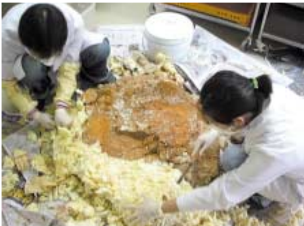
Photo 2. Removing of urethane form
