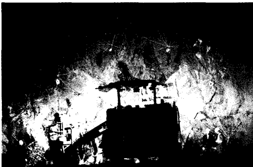
Fig. 5. Whole view of tunnel face(STA. 2+406)
