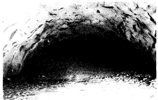
Fig. 11. Shotcrete laying at collapse point
