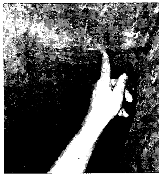
(b) Shotcreted ECC layer
