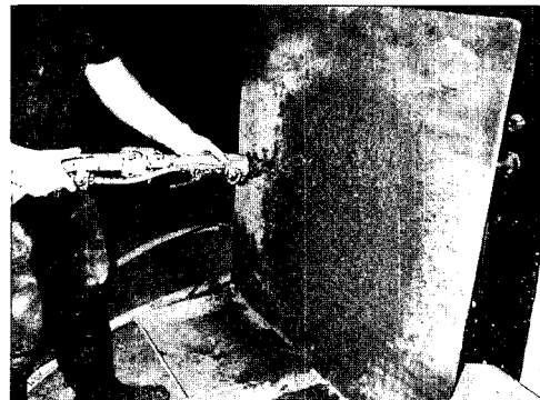
(b) Spraying process on a vertical surface
