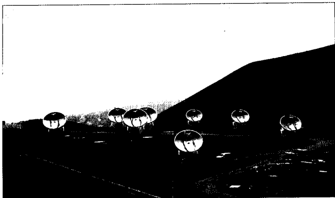
Fig. 1. — The completed SMA. The transporter used to move antennas is also shown in the right side of the foreground.
