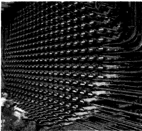
Fig. 1 Feeder pipes in PHWR reactor
