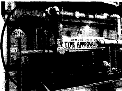
Fig. 1 Installed SCR system in HiMSEN engine
