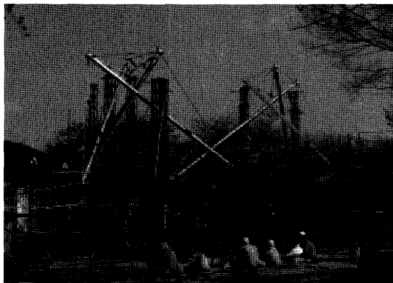
(c) Two three-strut tension systems
