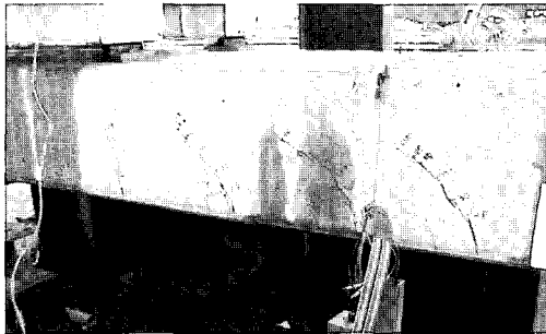
Fig. 7 Cracks view of rectangular beam RB1200
