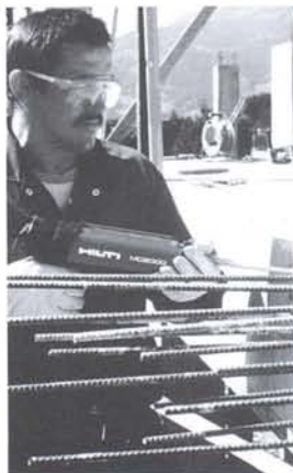
Fig. 12: Hilti HIT adhesive mortar being injected into rebar holes.
