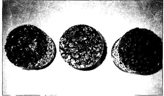
그림 7. Debonding between the waterproofing membrane and the concrete (Liquid systems)
