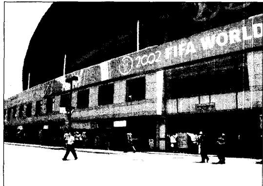
Figure 14. The stadium commercial area for 4 season use: after construction
