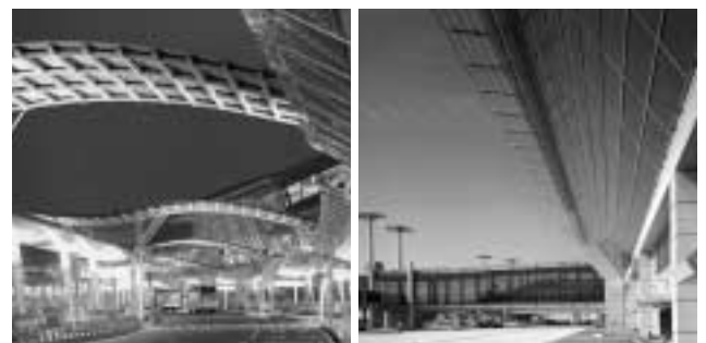
Fig. 3 Exteriors of the Incheon Passenger Terminal
