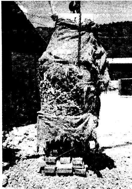
Fig. 7. View after Blasting, Column I (C+A)
