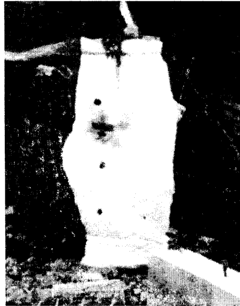
Fig. 8. View after Blasting, Column I (C+B)
