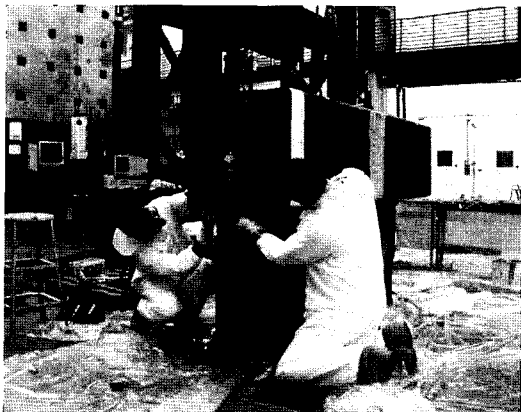
Figure 6 Retrofit of bridge cap beam with carbon fiber reinforced polymer sheet
