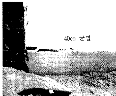
Fig 1. Coating crack found in field.
