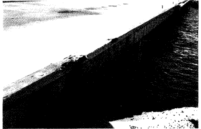
그림 1(b). Initial mechanical damage ; corrosion followed at jetty at St. Eustatius
