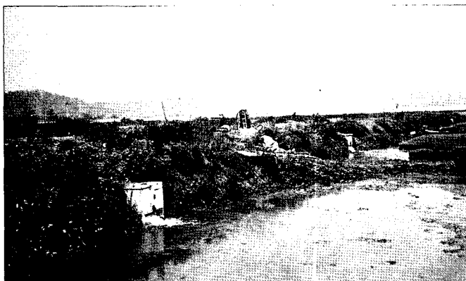
<Photo 2> Installation of semi-automatic inlet in field
