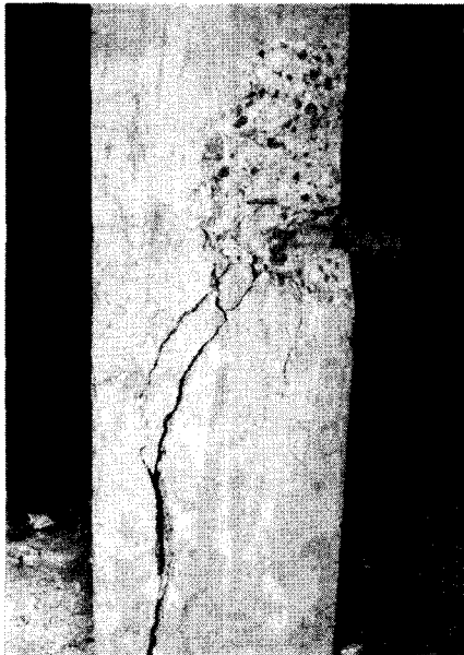
(c) Spalling of Concrete Cover
