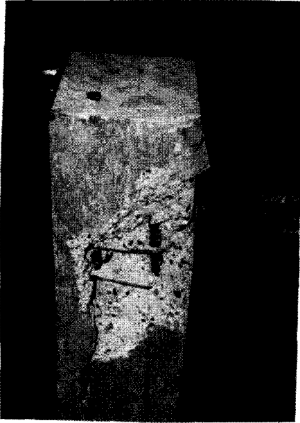
(b) Side Cracks
