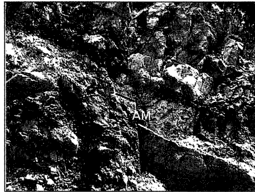
Fig. 11. A fault corresponds to the type III. AM; apparent dip separation.
