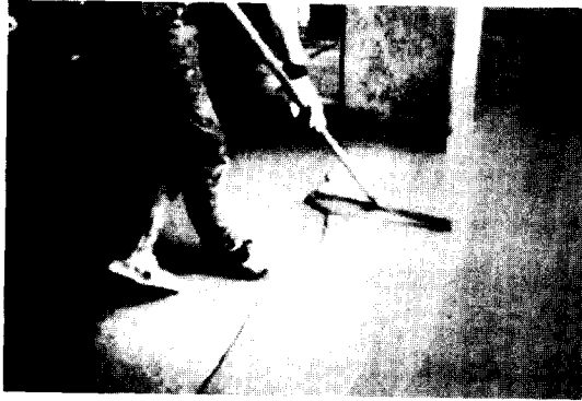
Fig. 6 Application of Elastomeric deck coating on the parking slab
