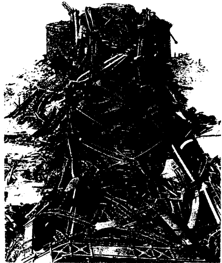
Fig. 4 The collapsed Quebec Bridge [17]
