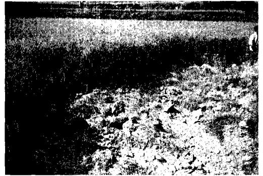
Photo 2. III type (inside paddy) collapse
