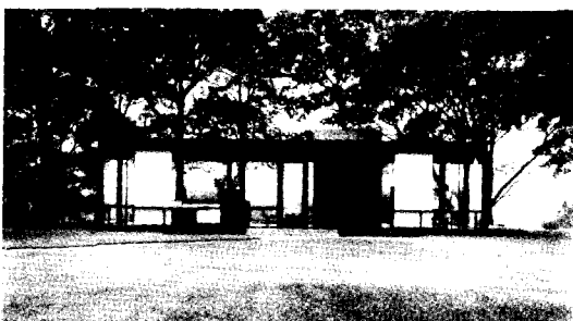
Figure 9. Philip Johnson house, New Canaan, Connecticut. All exterior walls are glass, creating an open effect comparable to a Japanese house. The simplified ground plan resembles the Japanese modular system (Frampton, 1985, p. 241).
