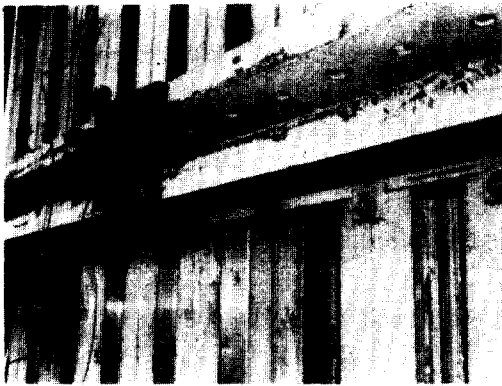
Fig. 5 Form details at ties.
