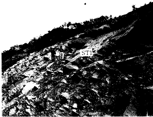
Fig. 4. Planar failure directed to slope front face by major fault.
