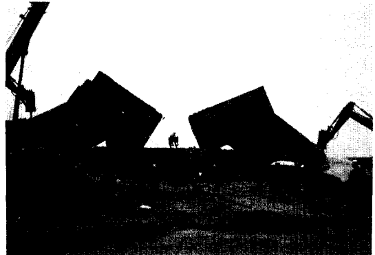
R.C partition after sawing
