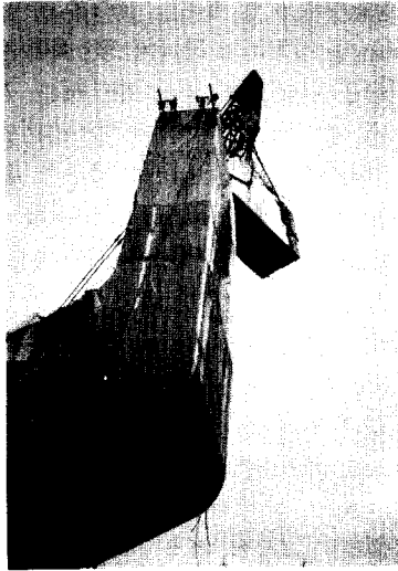
Downward movement of Reinforced concrete
