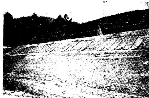
fig 2. View of slope experiment site at Dankook Univ. Chun-ahn campus.
