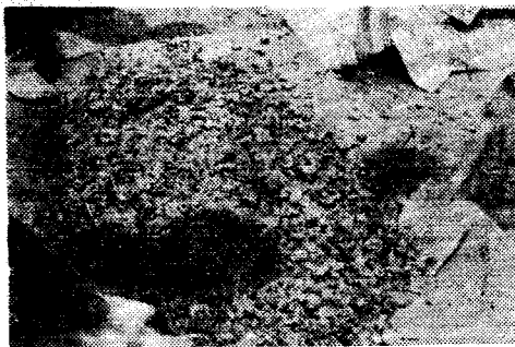
Fig. 4. Mixing for Steel Fiber Concrete
