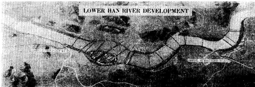
Fig. 6 Location of Submerged Weirs
